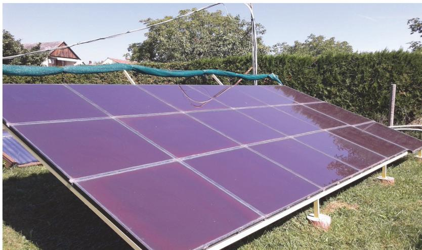
*Fig. 5.* The 11-year-old amorphous silicon solar panels
