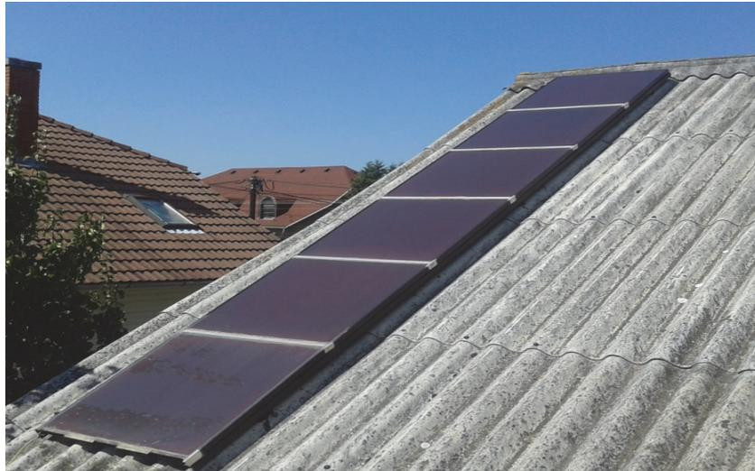
*Fig. 6.* Amorphous silicon solar panel on the roof.
